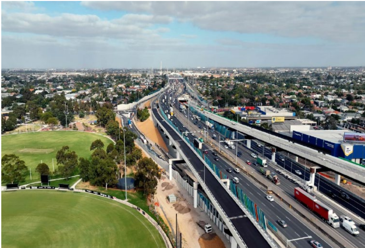
Figure 3: West Gate Freeway looking west (WGTP image)
