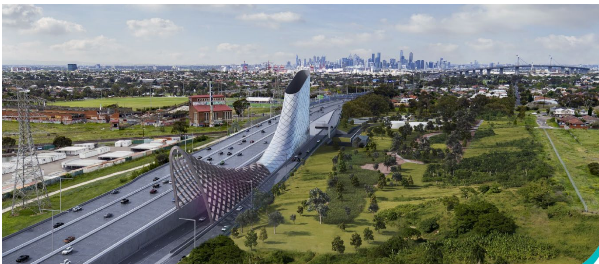
Figure 5: Future Southern Outbound Tunnel Ventilation Structure (WGTP image)
