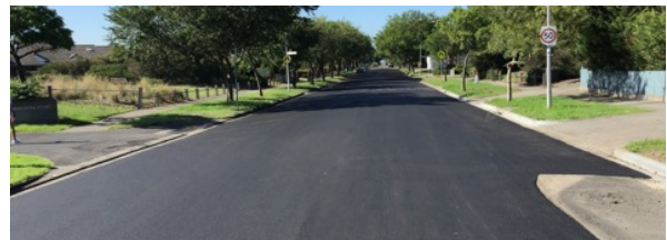
Dohertys Rd Resurfacing
