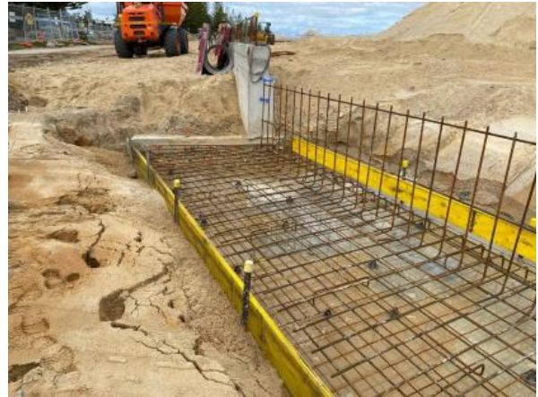
Image: Altona Beach Entry works underway
