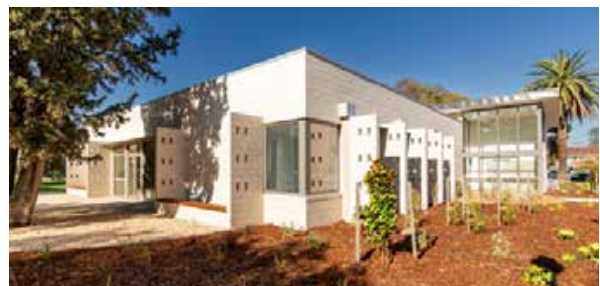
Dennis Reserve, Williamstown - Multipurpose Pavilion
