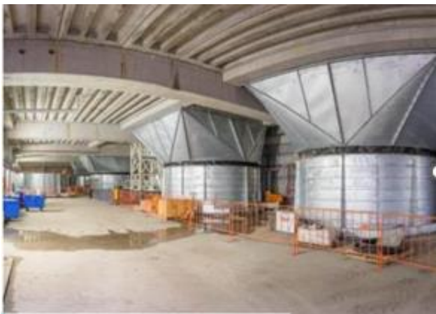
Image: View from inside the ventilation structure
