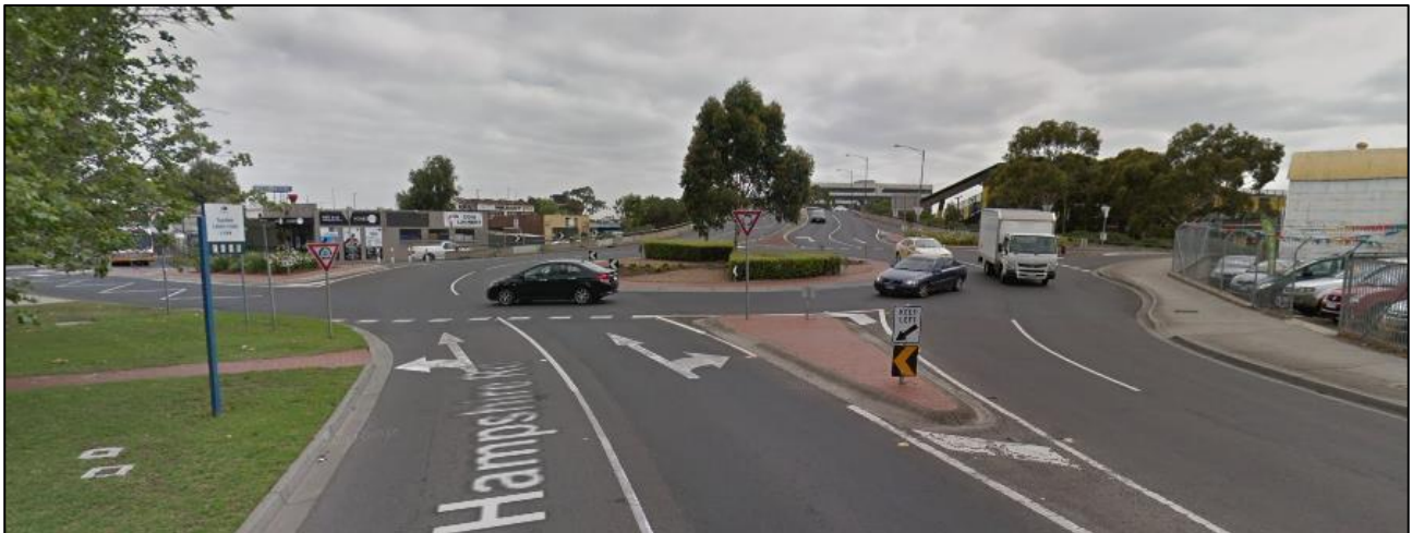
Roundabout (City of Brimbank)
