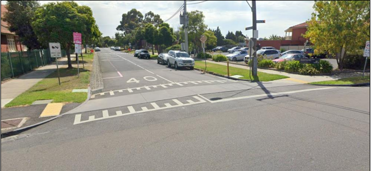
Raised Threshold Treatment (City of Moonee Valley)
