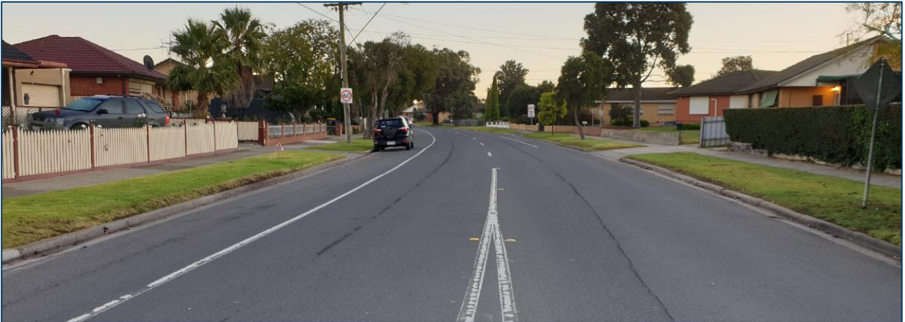
Figure 4-4 Bladin Street, looking north near Hillman Street
