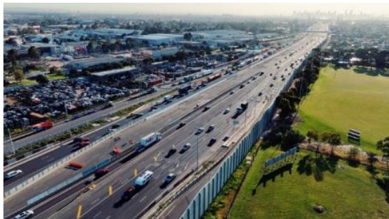
Image: West Gate Freeway widening works looking east from Grieve Parade
