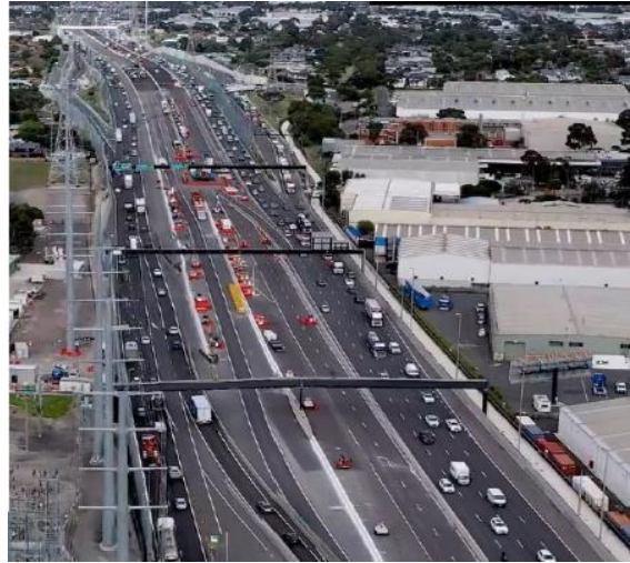
Image: West Gate Freeway West Zone Works - Outbound
