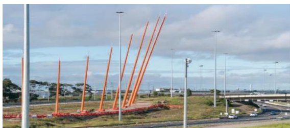
Image: Feature lighting at the M80 interchange
