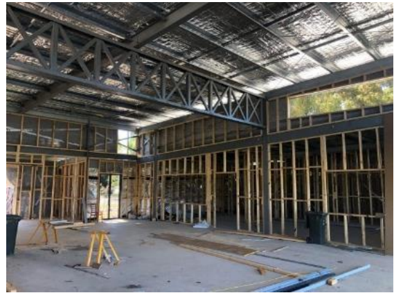
Image: Kim Reserve pavilion works
