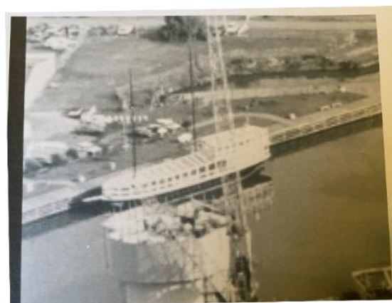
Image: Lighters (barges) after the Explosives reserve had ceased operations
