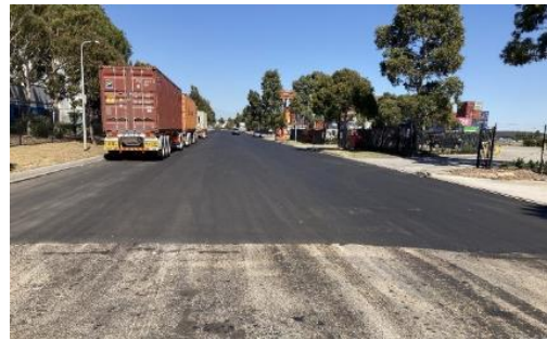
Image: Newly laid asphalt base course at Toll Drive
