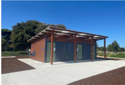
Image: Public Toilet block at PA Burns Reserve
