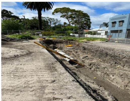
Image: Drainage being installed in Melbourne Road Williamstown
